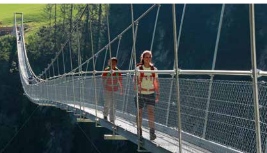
Pedestrian suspension bridge over the Höhenbachschlucht
